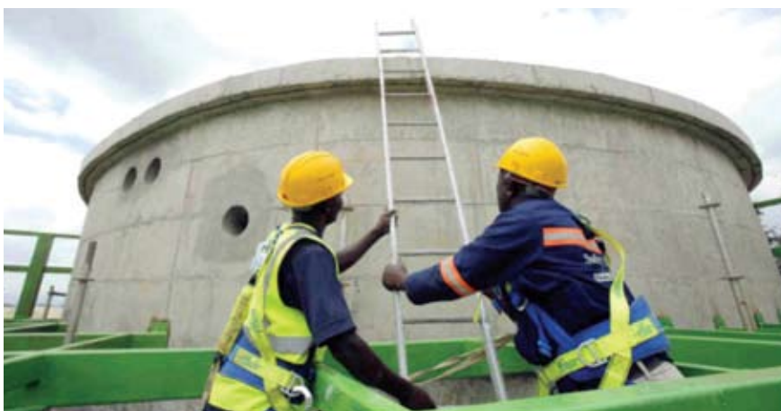
Biogas : Storage tank
