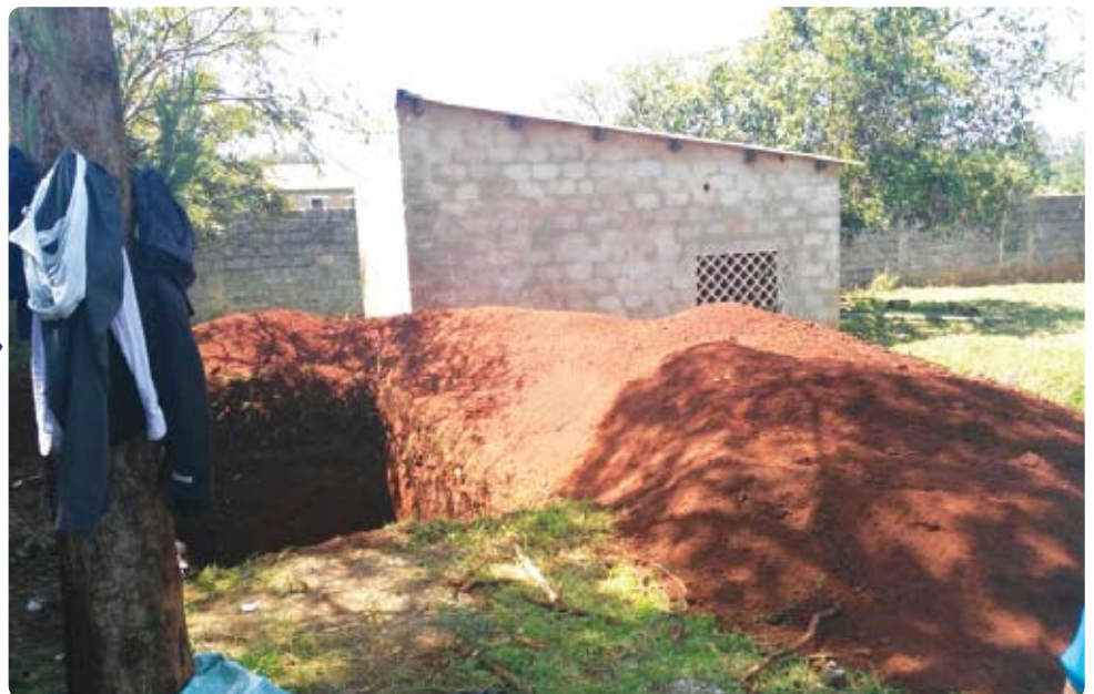
Project – sanitary building (Child Shelter, Ngong)
