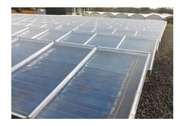
only kerosene was used. Currently, Stokman uses the 'free energy' of sunlight, which warms the water up. This hot water is stored in a completely isolated heat storage tank. With this heat, the greenhouse gets warmed up at night. "Earlier, Stokman sometimes used 1400 litres of kerosene a night! Currently, it uses a maximum of 400 litres. A confirmation of the saving of 1000 litres per night! According to Stokman Rozen Kenya Ltd. the period of return on investment for this project is two years!"
